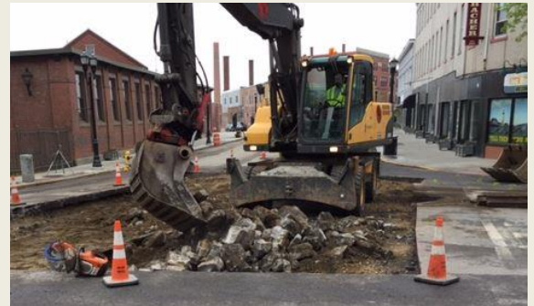
Top: Digging and preserving original cobblestone
