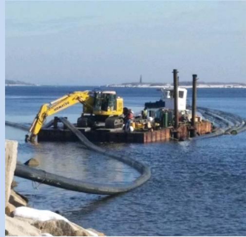
Mechanical dredging of the Saco River Federal Navigation Channel began on Saturday, February 9. Mechanical dredges work by digging up or gathering sediment from the bottom surface of a body of water. Sand from the westerly end of the river that is mechanically dredged will be brought to the deep scour hole mid-river for disposal.
